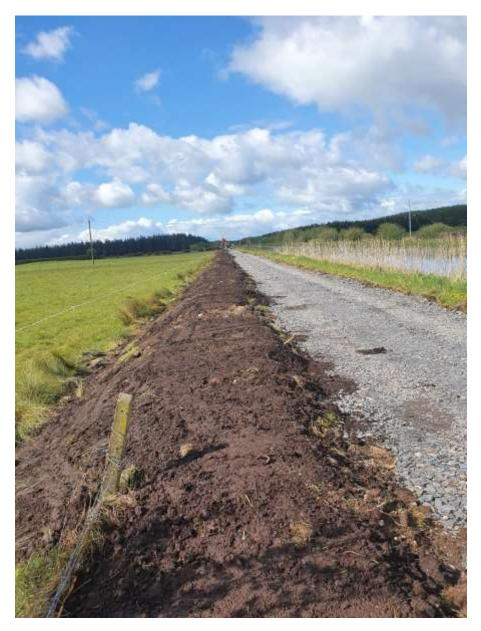
Fig2 – Taken at CH9200 looking South. Embankment, excavation terram & stone base laid.
